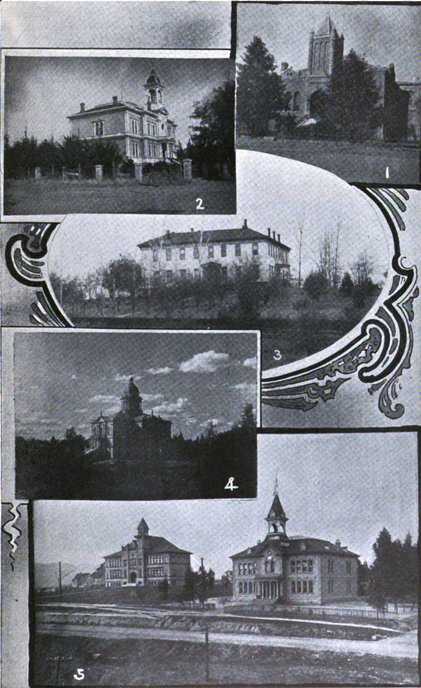
PUBLIC BUILDINGS. —1. Hall of Records, Yolo County. 2. Convent at Colusa. 3. High School, Placer County. 4. Court House, Placer County. 5. High School left, Grammar School right, Vacaville, Solano County.
